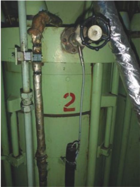
TCS-01CA-PMI sensor installed on a MAN 6S60 ME two-stroke diesel engine
